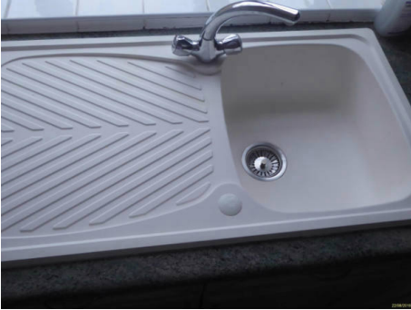
Sink - light marks in base
