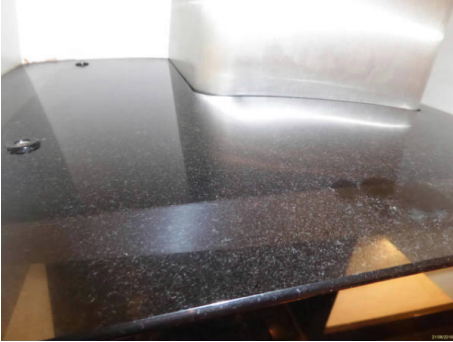
Hood casing dirty
