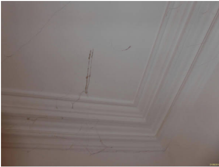
Cobweb strands on ceiling
