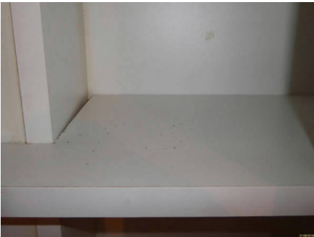
Units not clean
