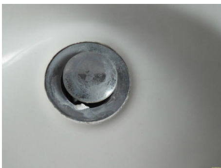
Basin waste not clean
