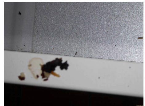
Units not clean
