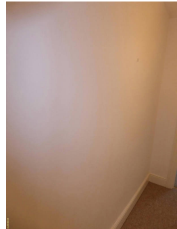
Landing mid level to bed 1
